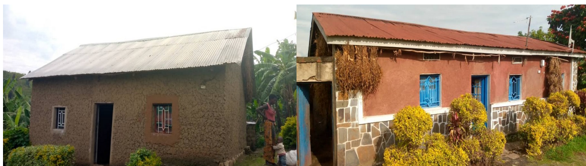
Figure.: Houses to be destroyed during implementation of the project
