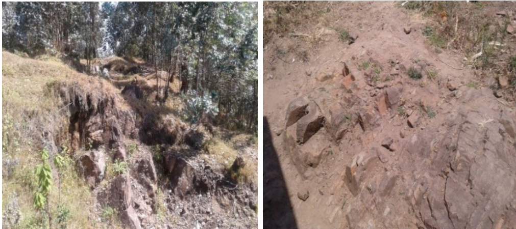
Figure 5: Rocky Based sites in the area which may serve as the foundation for the Construction of Storage Reservoirs
