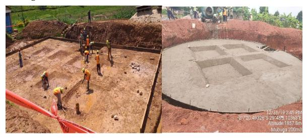
Picture 1: [above] Rebate fixing at a bottom slab of Mpanga 500m³ Reservoir and Picture 2 shows a casted and cured bottom slab of Mubuga 200m³ reservoir.
