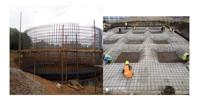
Picture 1 [above] shows steel works at **Gihuma WTP 200m³** reservoir and picture 2 shows the steel works on the bottom slab of **Nkomero 1000m³** reservoir
