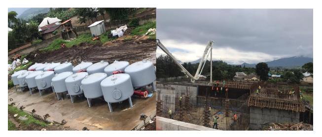
The Omni Filter System (OFSY) filters are already installed in their positions (picture1) and concrete casting works for the left side shear walls of the 6000m<sup>3</sup> Reservoir and its valve room (picture 2)
