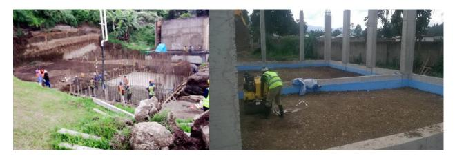
The raft foundation concrete casting for the valve room of 2500m<sup>3</sup> RWAZA reservoir are complete and the shear walls re-bars installation are ongoing. Photo 2 is the backfilling and compaction of chlorine and Chemical building.
