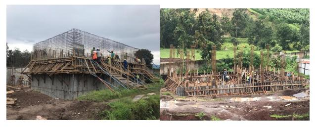
Picture1: 6000m³ reservoir valve room ready for the second casting while the shear walls of 1.8m for the chemical Chlorine building was ready for casting as shown by picture#2
