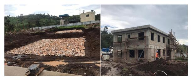
Picture 1: The excavation works for the clarifier and sedimentation are completed.
