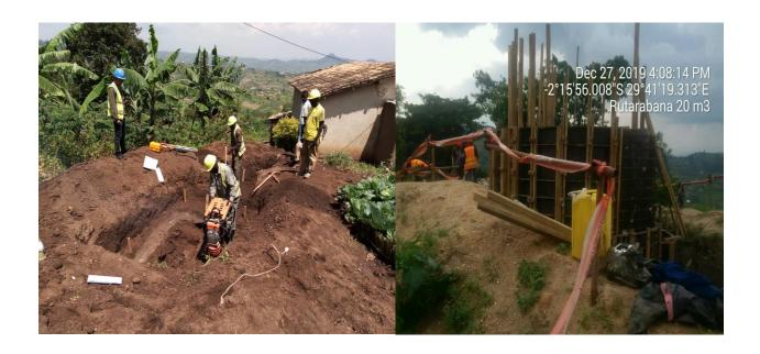
Picture 1 [above] shows excavation on a site to be constructed a water kiosk in **Ruhango** and picture2 is about fixing formworks on **Rutarabana (Gitwe) 20m³** reservoir.
