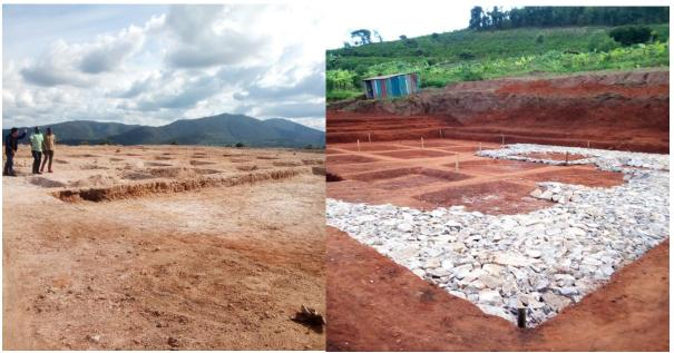
Picture 1 and 2 show site camp installation, photo3 shows Clearing, Excavation, levelling, setting out, DCP, access road for Kanazi 2000m³ reservoir location while picture number 4 shows hard core laying at 1000m³ Sovu reservoir.
