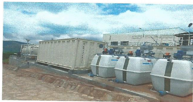
Water treatment compact units at Gihuma (Muhanga) and Cyondo (Nyagatare)
