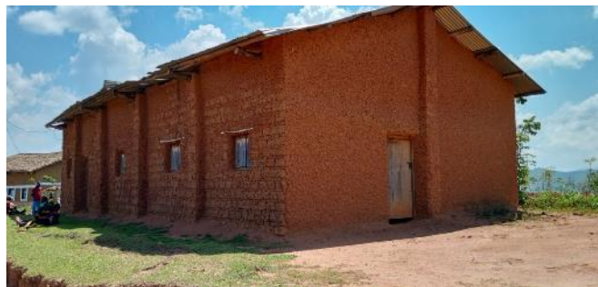
Figure 19: Main building-ADEPR MUHAMBARA
