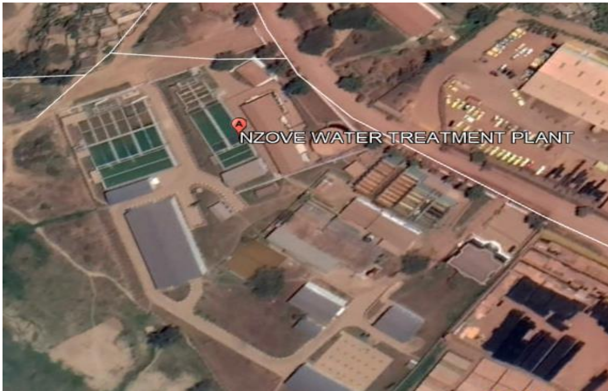
Figure: Nzove WTP complex is located in mixed land used area
