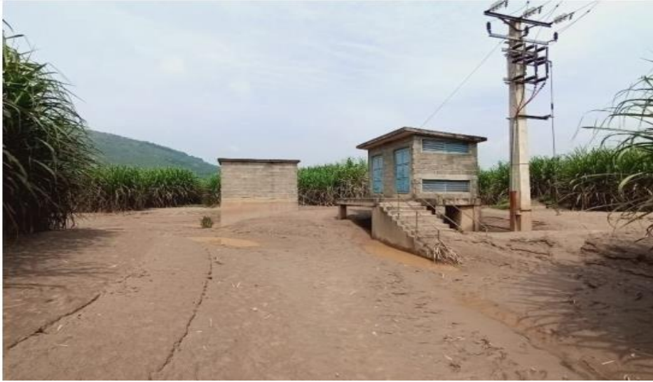
Figure: Electric line to be supplied to new borehole for raw water pumping and to other facilities
