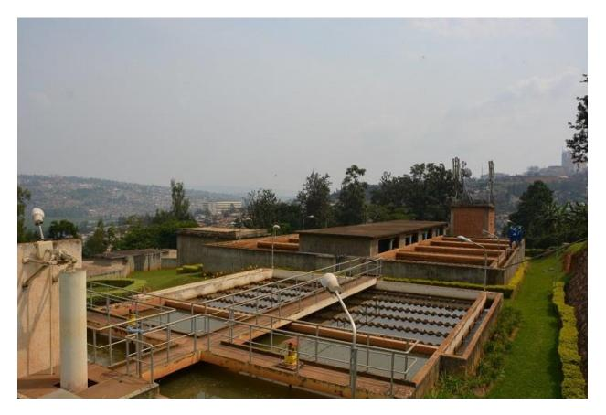
Kimisagara Water Treatment Plant supplies clean water to City of Kigali. It is located in Kimisagara cell, Nyarugenge District and is one of the three water treatment plants supplying the city dating back to the 1980s. It produces 29,000 cubic meters daily. Five pumping pipes transport the water to three pipes from the plant to reservoirs.
