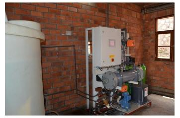
The treatment process is complex consisting of a mixture of at least three different chemicals to ensure good quality water. The plant makes its own chlorine and this ensures good quality/quantity of the chemical. This is imperative because the water is raw. Once the treatment is complete, the water is stored in four reservoirs within the plant then its pumped out to outside reservoirs in different parts of Kigali.
