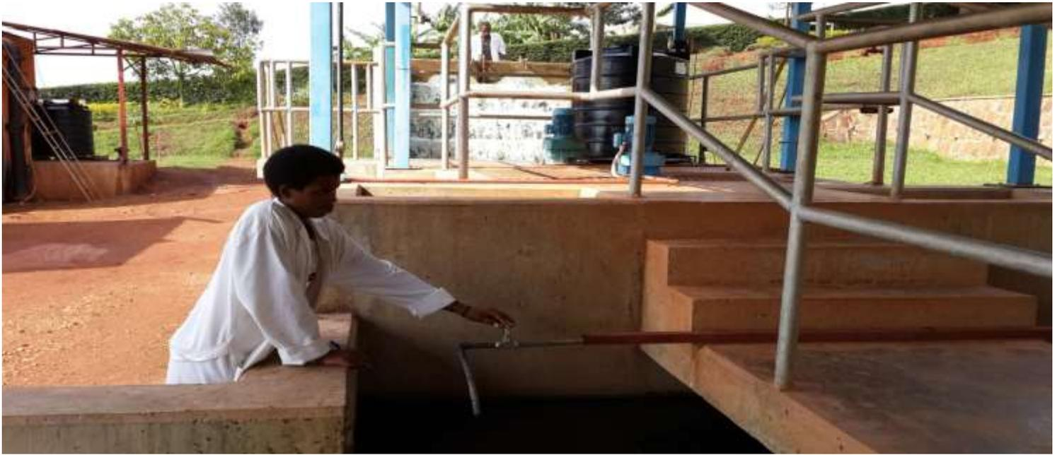
*Figure 5: Treatment chemical split dosing points*
